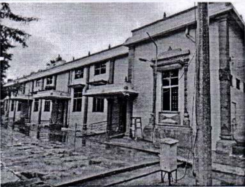
Auditorium under final stages of construction
